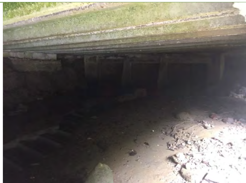
The 3 culverts (2000048193, 2000359099 and 2000671763) set back beneath parking garage.
