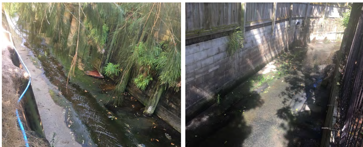
Figure 11: Typical examples of reaches in Management Zone 3. Concrete lined channels with timber bank lining on the upper reaches of the Glendowie Stream (GLE_TRIB4_9 left, GLE_TRIB4_5 right).
