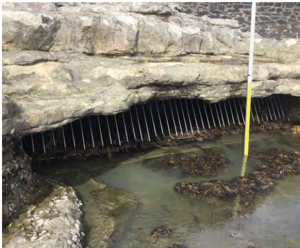
Auckland Council owned St Heliers coastal outlet with grill to trap debris is a partial barrier to swimmers and is likely to be temporal due to tides.
