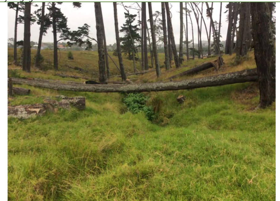
Modified channel with exotic cover of pine and no understory. Mass wasting of bank and incised channels.
