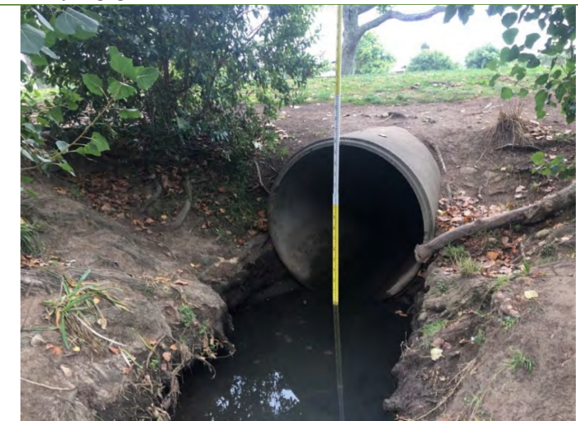
Asset ID 2000229311 with an unconstrained drop height of 1.6m close to the walking path.
