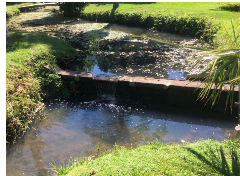
Weirs are complete fish passage barriers (GLE_MAIN_4).
