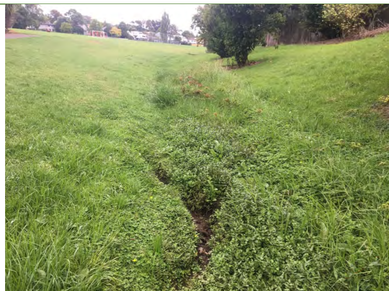
OLFP (Tributary ID: GLE_TRIB4_11) above the piped channel.
