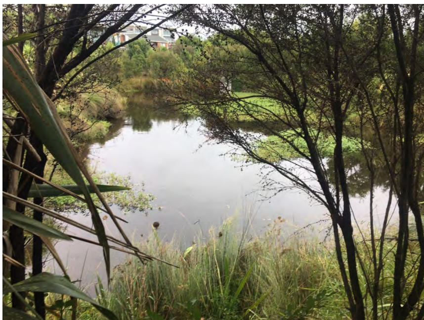
Figure 24: Wet stormwater detention pond, in the Glendowie catchment.
